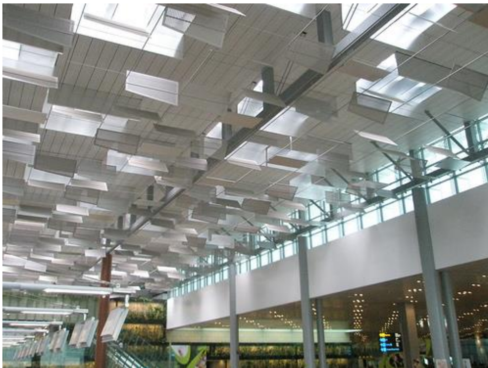
Figure 227: Daylighting System In Changi Airport Terminal 3
