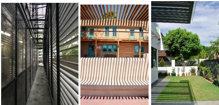
Figures 117, 118 And 119: Overhead Louvres Used Internally And Externally
