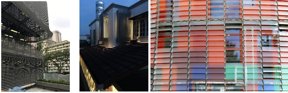
Figures 114, 115 And 116: Metal Louvres Providing Shade And Glass Louvres Providing Visibility. Both Allowing For Ventilation
