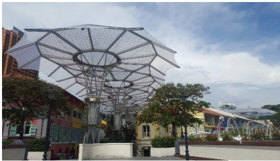
Figures 130 And 131 ETFE Roof Canopy At Clarke Quay, Singapore
