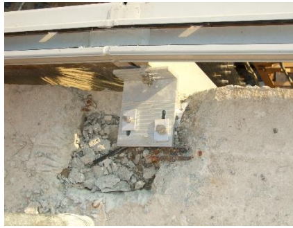
Figure 37 Extruded Aluminium Glazing Frame Figure 38 Extruded Structural Aluminium Bracket
