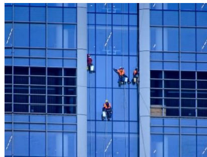
Figure 113 Use Of “Spider Man” For Maintenance
