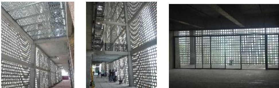
Figures 124, 125 And 126: Use Of Air Block In PJ Trade Centre
