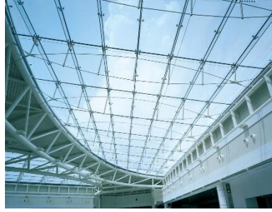
Figures 62 And 63: Cable-Net System (Detail And General View)
