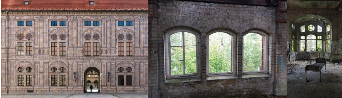
Figures 4 And 5 Windows Placed Adjacent To Each Other To Give An Illusion Of A “Larger Window” (Courtesy: Pixabay.com)
