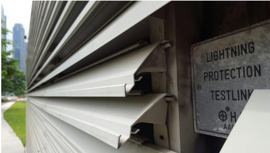
Figure 120: Water-Tight Louvres (Courtesy: Patricia Collera)
