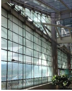
Figures 62 And 63: Cable-Net System (Detail And General View)
