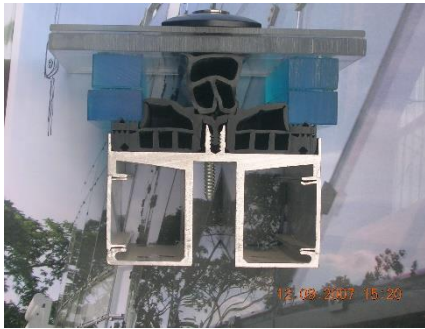
Figure 37 Extruded Aluminium Glazing Frame Figure 38 Extruded Structural Aluminium Bracket
