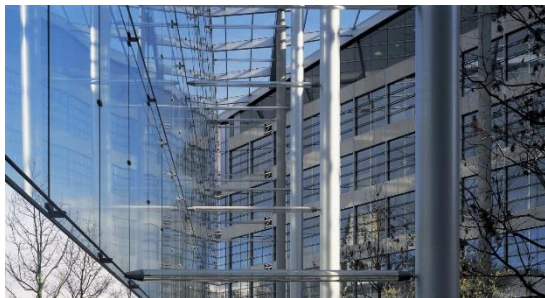
Figure 68 Glass Tubes As Compression Struts (Courtesy: Foster + Partners Pte Ltd)
