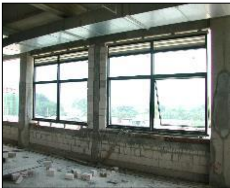
Figure 34 Stick System Under Installation
