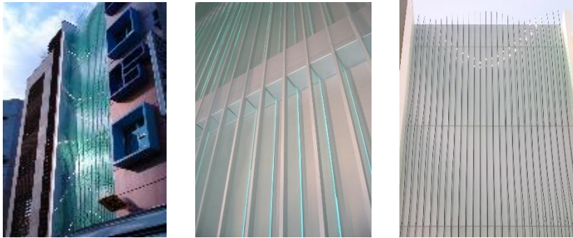
Figures 45, 46 And 47 Glass Fins With Aluminum Insulated Panels
