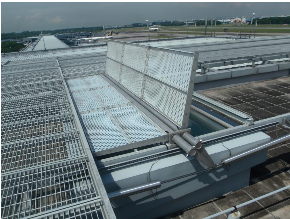
Figure 229: Rooftop Installation Of Daylighting System In Changi Airport Terminal 3
