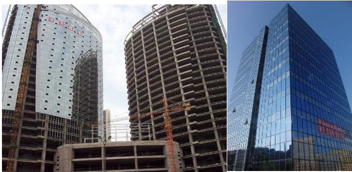
Figures 26 And 27 Unitised System Used On High Rise Buildings
