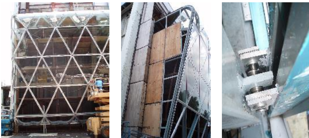
Figures 165, 166 And 167 Performance Test Assembly (Courtesy: Arup Singapore Pte Ltd)
