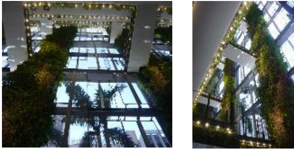
Figure 50 And 51 Layered Glass Façade Allows Air And Drizzles In For The Plants
