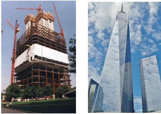
Figures 28 And 29 Unitised System Under Erection And Completion (Courtesy: Fosters + Partners Pte Ltd (Fig 28) and Pixabay.com (Fig 29))
