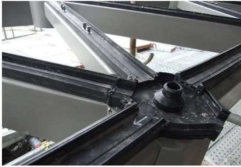
Figure 39 Extruded Gaskets (Courtesy: AgFacadesign & G Facadesign Pte Ltd)
