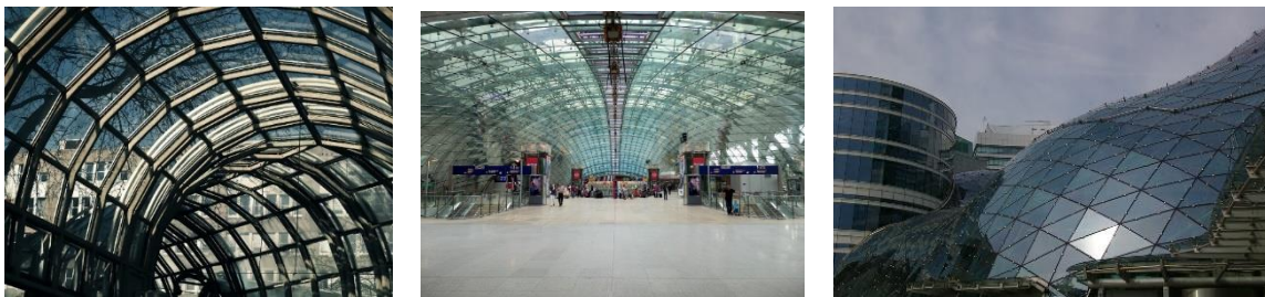
Figures 42, 43 And 44 Monocoque Structures Used On Different Sites And Support Systems
